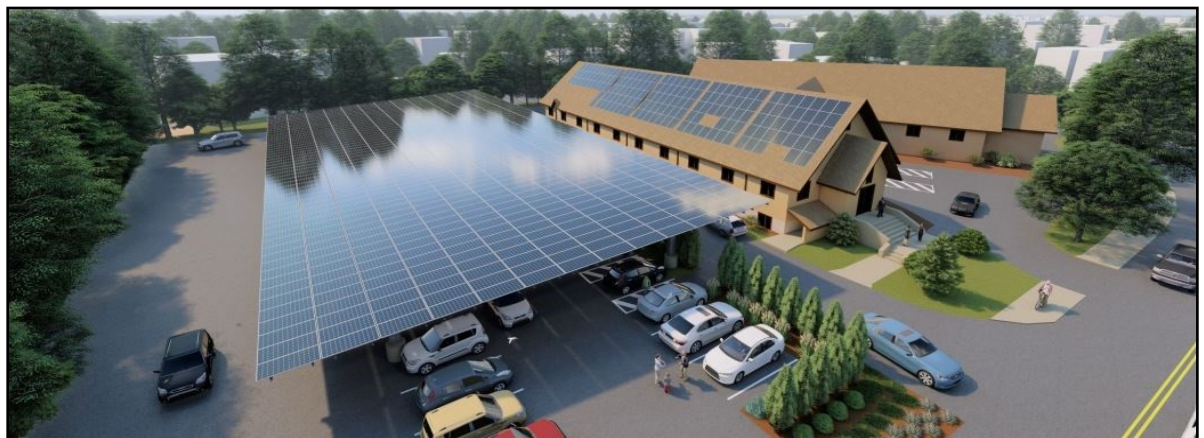
Our newly installed solar canopy
