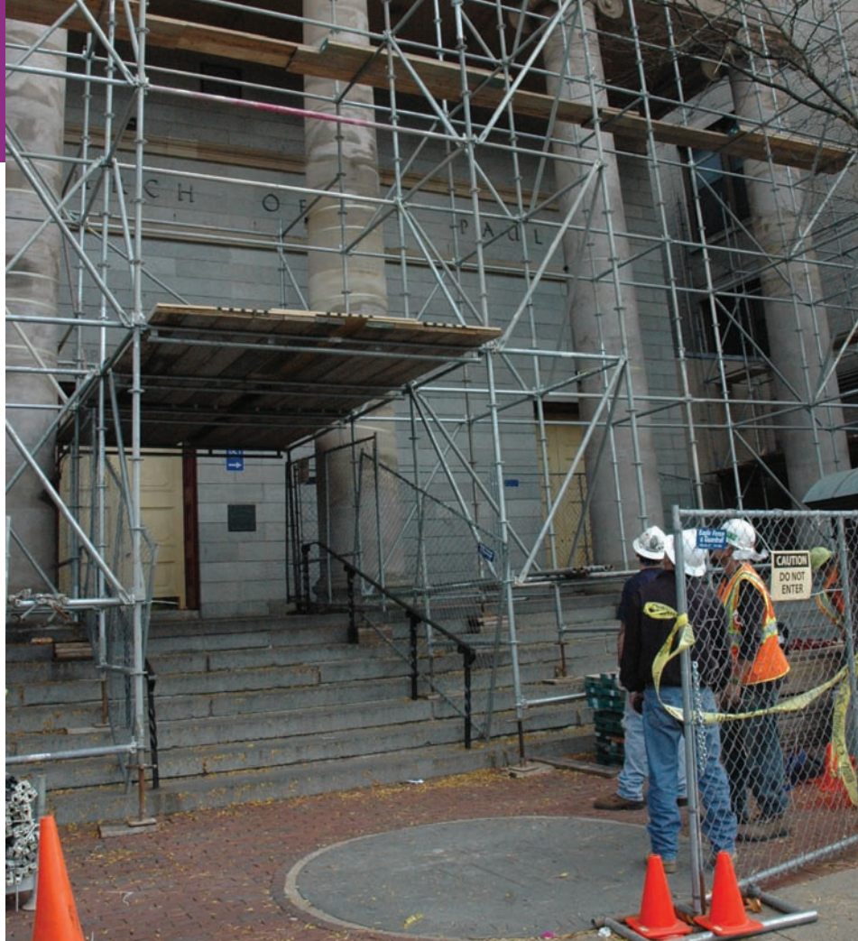
Repair work on the cathedral church's façade was completed in the fall to prepare for the pediment sculpture installation this spring.
